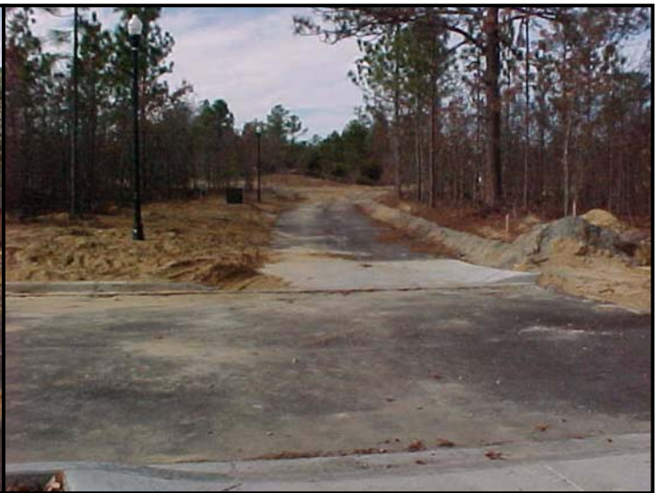
Looking west from site toward commercial area
